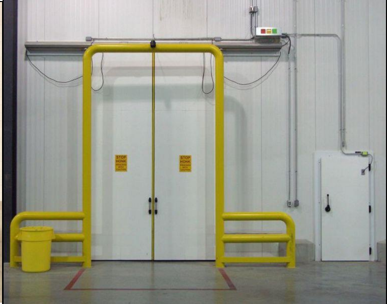
Cold Storage Doors
